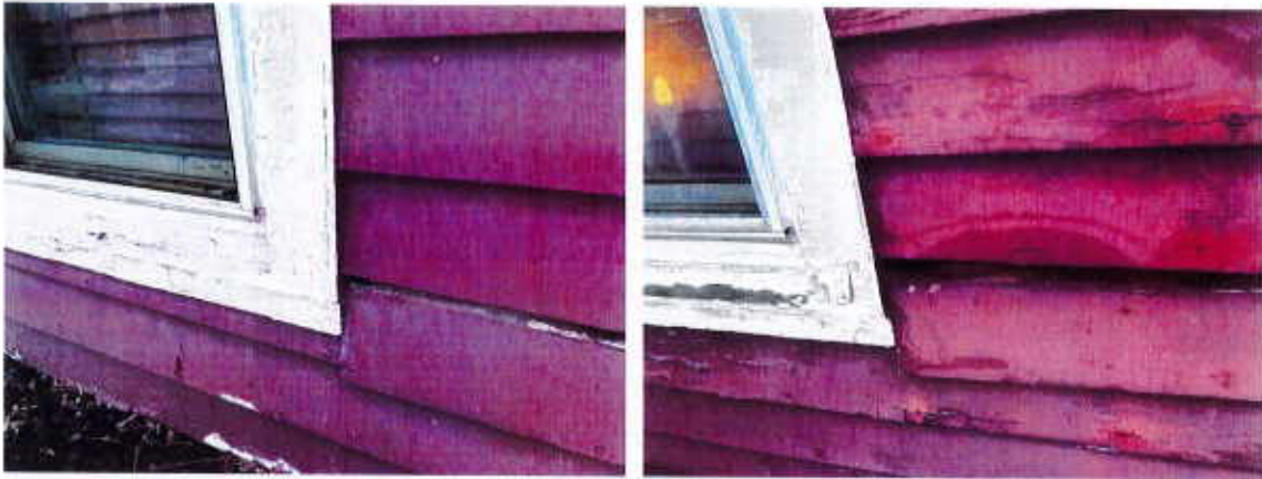
Examples of loose siding boards.
