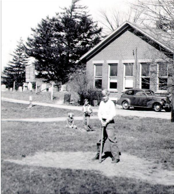
In this circa 1940s image, the cemetery at Bushnell's Basin is visible just behind the District 1 School. The building was demolished in 1978, after heavy snows collapsed the roof.
