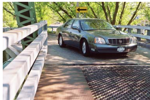
Pedestrian's view crossing from north to south on Marsh Road Bridge
