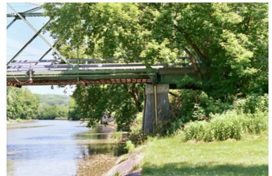
Southern abutment – Marsh Road Bridge
