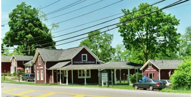
Canal Walk complex
