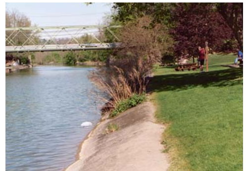
Sloped wall along southern Canal bank
