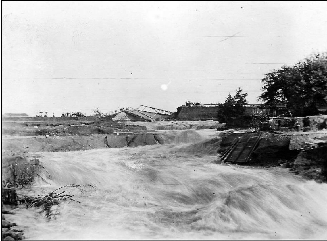
A view looking south at the collapsed Wapping Road Bridge on May 26, 1908. The western portion of Ayrault Road was once called Wapping Road. The bridge was replaced with a Double Warren truss bridge of steel construction the following year.
