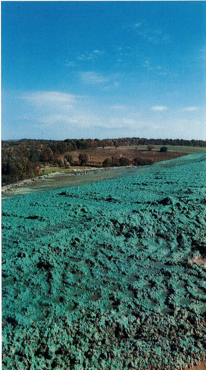
Photo 17: Northeast corner of cap after seeding
