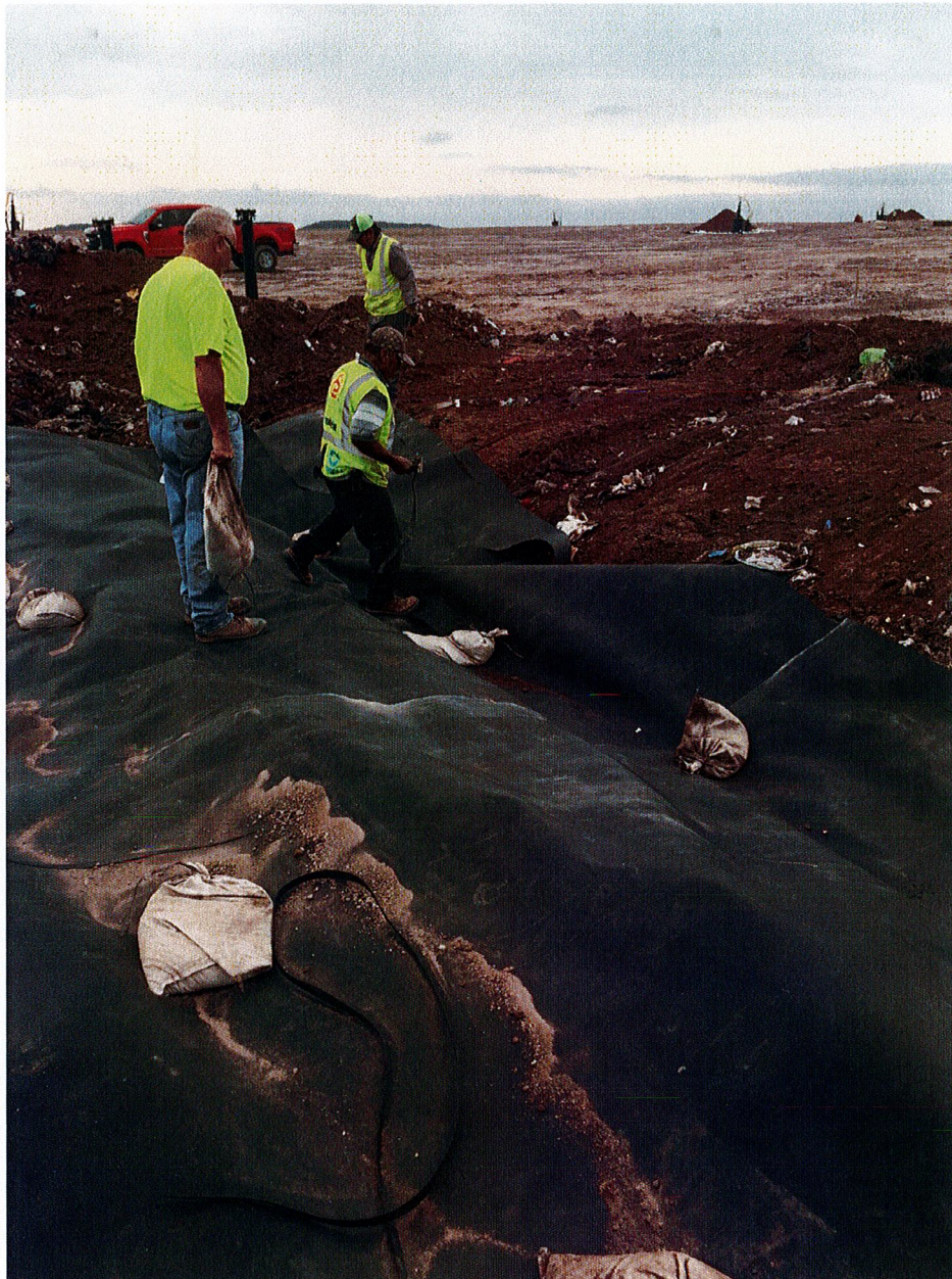
Photo 6: Welding liner for downchute on north slope of cap
