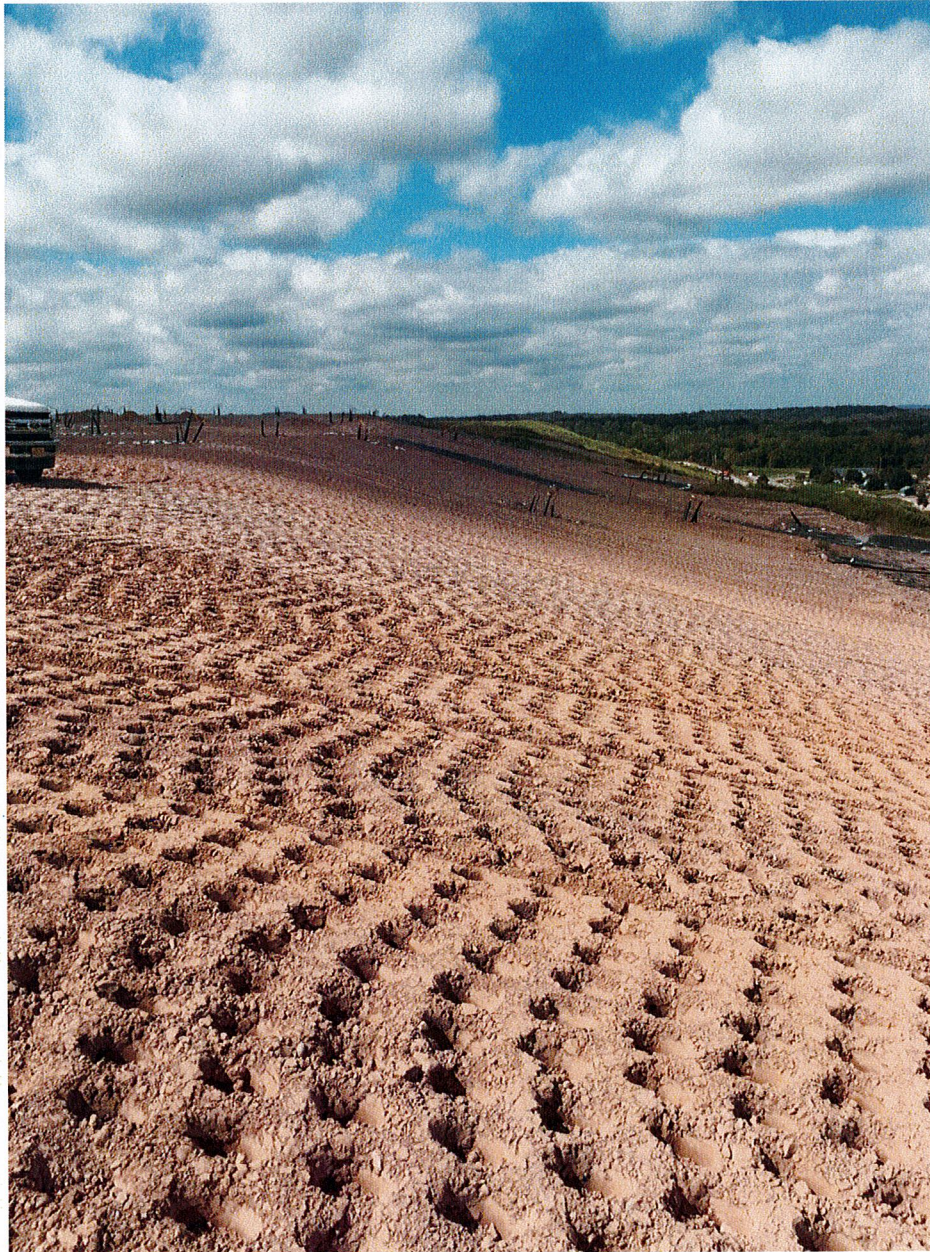
Photo 11: Completed second lift on north slope of cap area
