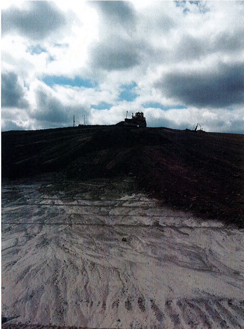
Photo 14: Grading lift one on east slope of cap area
