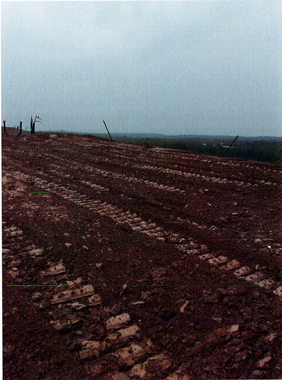
Photo 10: Lift one in northeast area of cap
