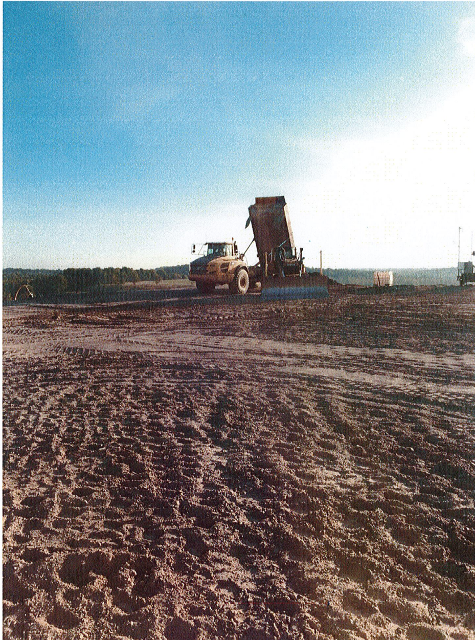
Photo 15: Placing topsoil on east slope of cap
