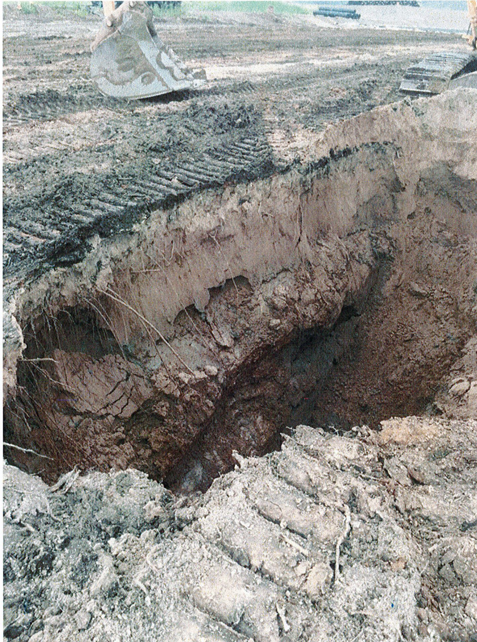
Photo 2: Test pit for cap material
