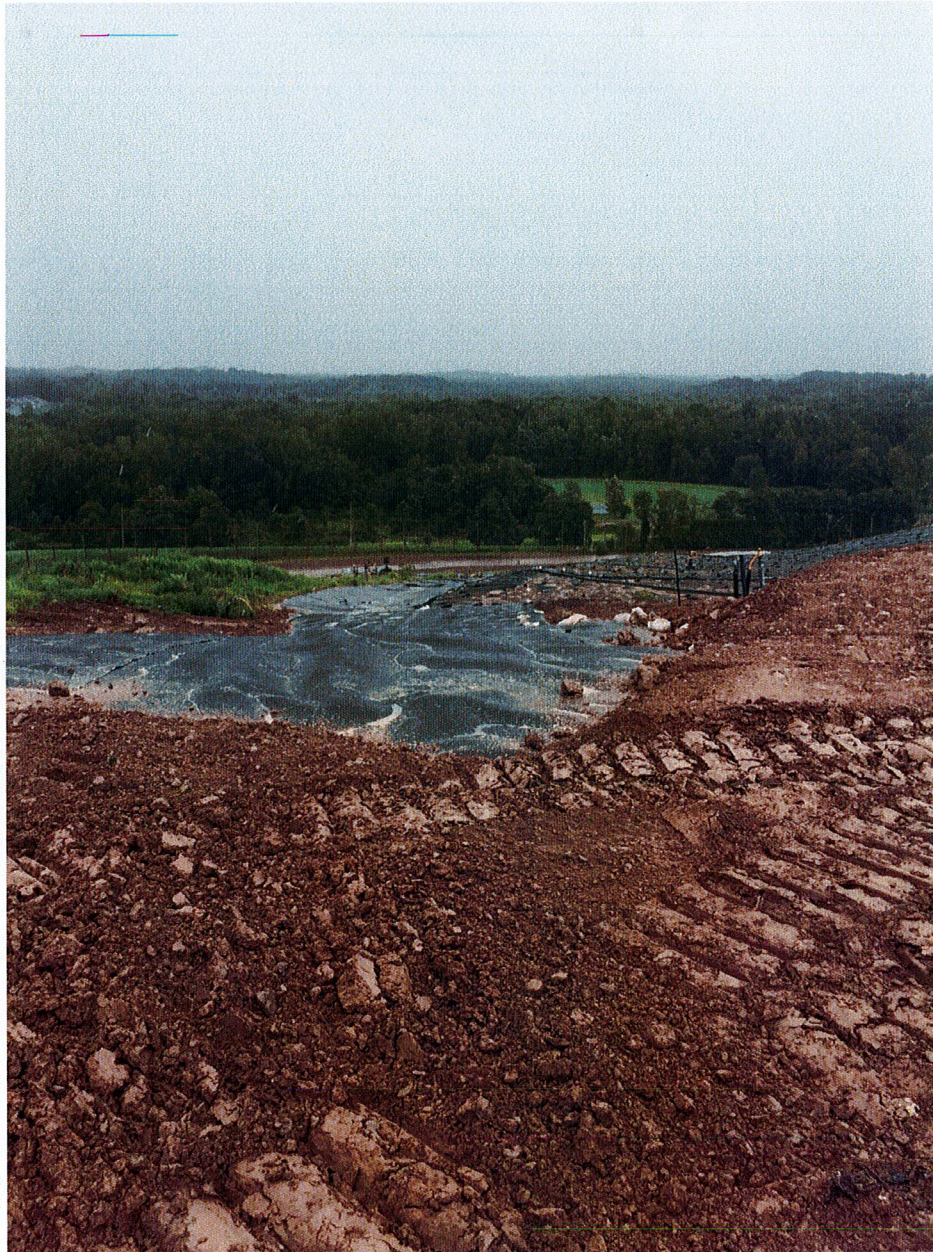
Photo 8: Completed downchute grading
