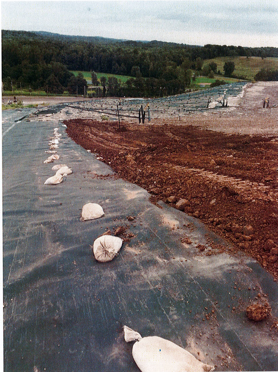
Photo 7: Backfilled anchor trench for downchute on north slope of cap
