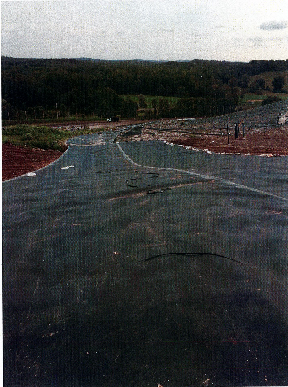
Photo 5: Lined downchute on north slope of cap area
