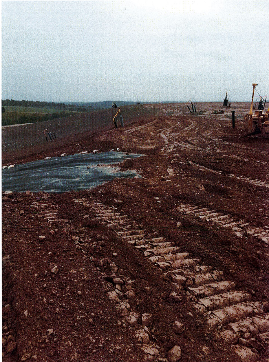
Photo 9: Completed downchute grading
