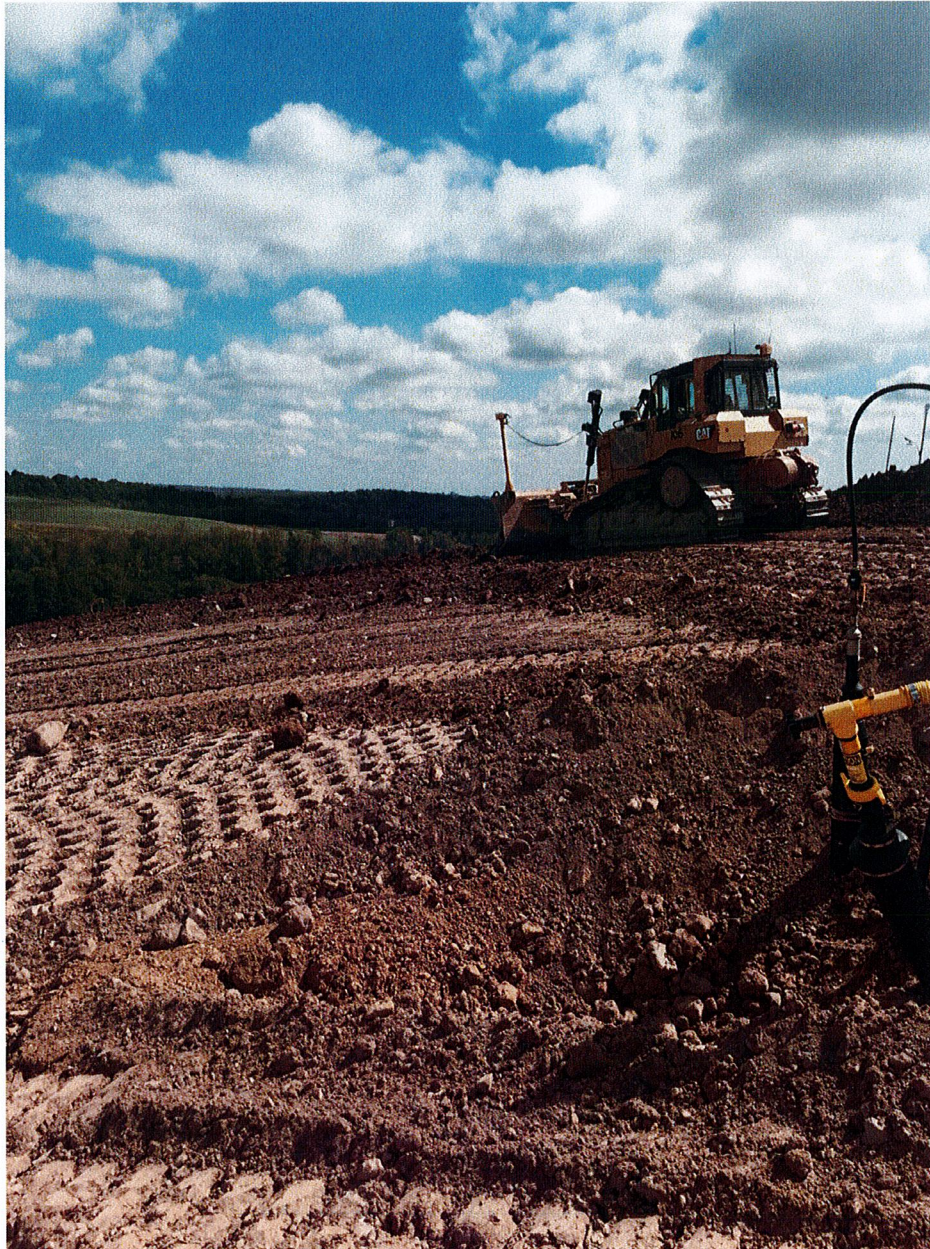
Photo 13: Grading lift 2 using GPS guided equipment.
