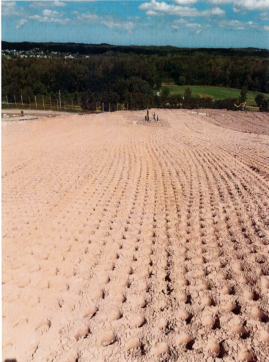
Photo 12: Second lift on north slope of cap
