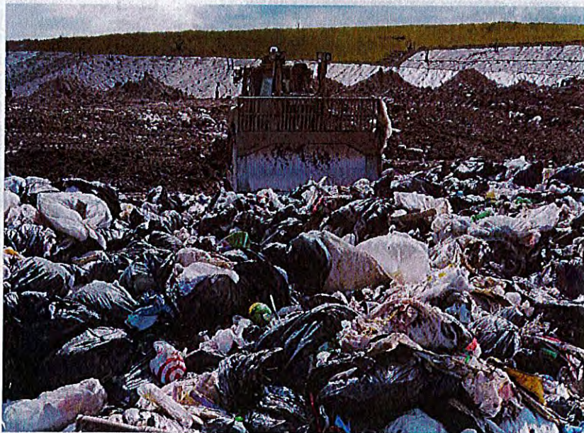
Photo 16 – Equipment Used to Spread Out Waste Pile Prior to Cover Soil
