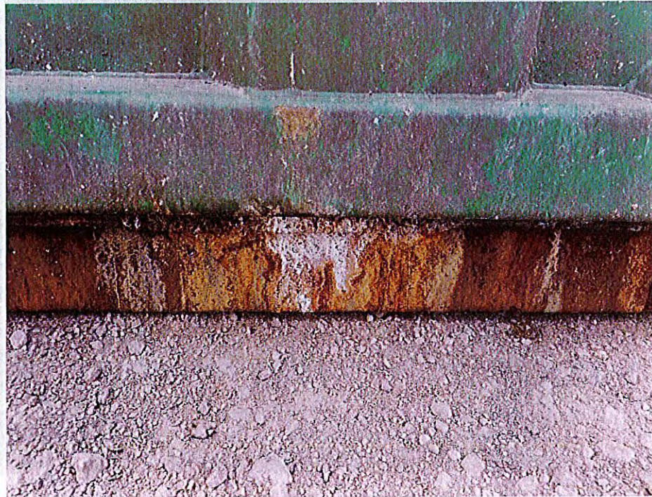
Photo 80 - Varick Rail Container WMNY #10410 - Bottom Left Door
