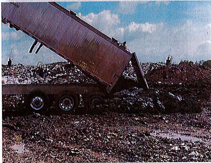
Photo 32 – Bio-Solids being unloaded in active area of Cell 12
