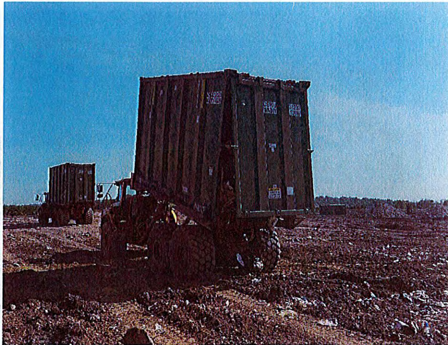
Photo 95 – Varick Rail Container WMNY #10999 ready to be unloaded in Cell 12
