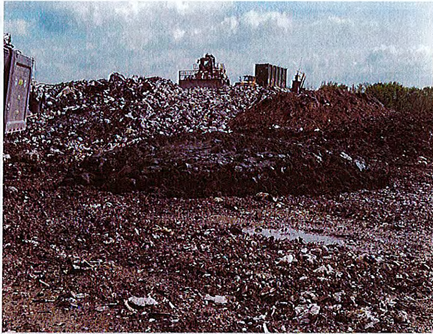
Photo 33 – Bio-Solids Pile in active area of Cell 12
