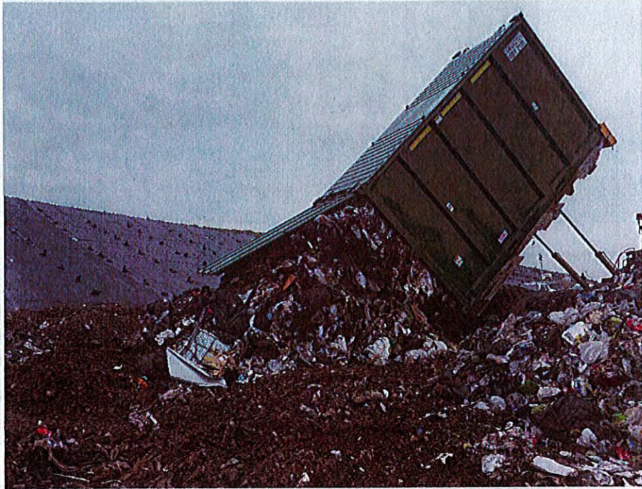
Photo 125 – MTS Hamilton Rail Container WMNY #2109 being unloaded in Cell 12
