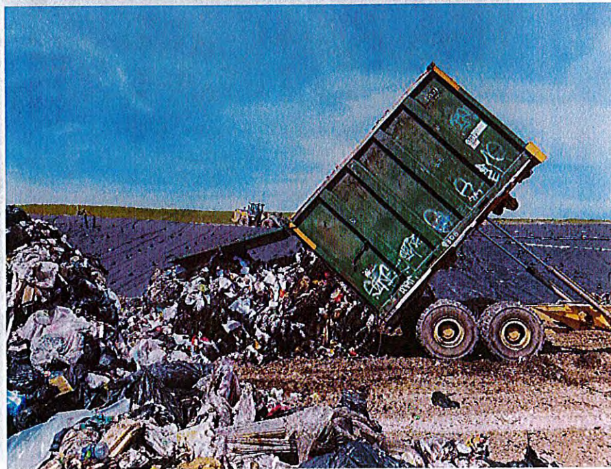
Photo 70 – Review Rail Container USWX #9305 being unloaded in Cell 12
