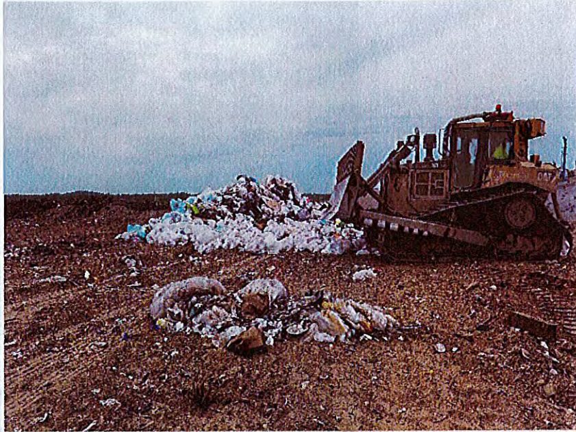
Photo 27 – Equipment used to spread WM Local Front Loader Waste Pile
